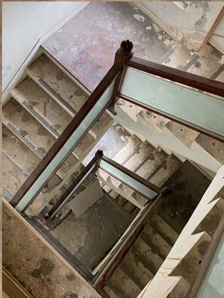
● Spiral Staircase | New Seminary Dormitory
